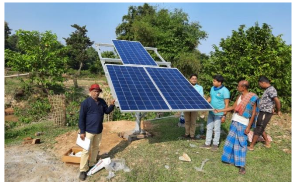
Solar pump being installed in Daspara, Charilam block in Bishalgarh sub-division
