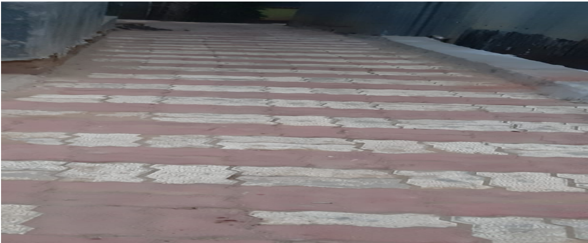
Paver Block Road at 79 Tilla under AGCL
